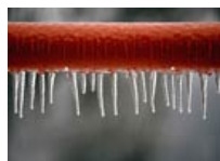
Anti Freeze Winterize your home's plumbing
